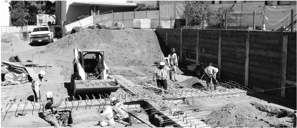
The construction crew works throughout most school days. LEO OSTROY HARP
